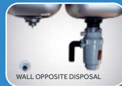
WALL OPPOSITE DISPOSAL
