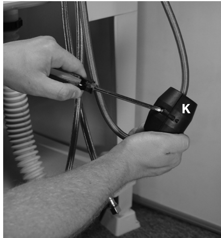
13 Attach the counterweight (K) to the faucet line. Position the counterweight at the lowest point of the line. Adjust as need.
