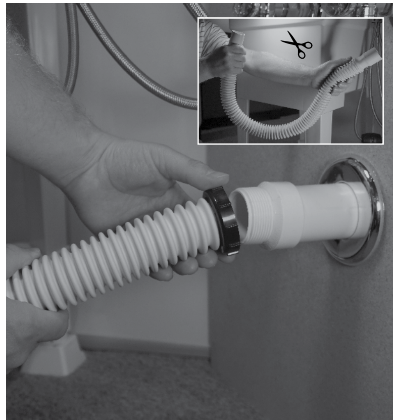
16 Measure the Simple Drain® tube so that it makes a trap as shown in Step 17 and cut to length. Thread Simple Drain® to the drain line by hand until snug. DO NOT use a wrench. Note: it can be installed as an S-trap as well.
