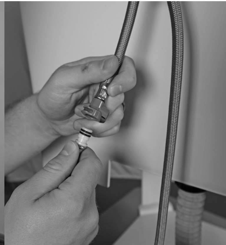
14 Push together the faucet quick connect lines.
